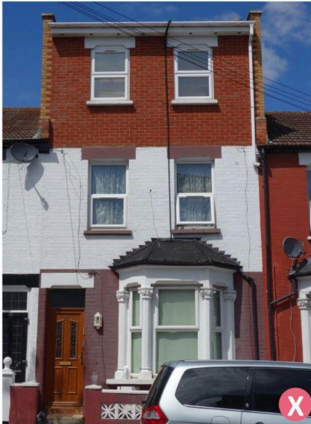
Fig.24: Roof extension is not acceptable due to change in materials that draws too much attention on the upper element
