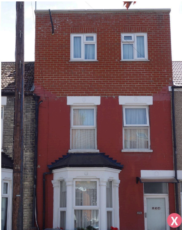
Fig 29. The roof extension windows are not in keeping with the existing window shape, size and alignment.
