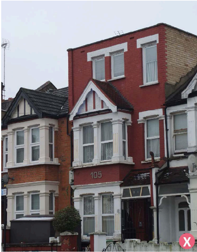
Fig 30: The roof extension is bulky and detracts from the front gables architectural character. The pitched roof form has been lost and the flat roof is not in keeping with the neighbouring properties.
