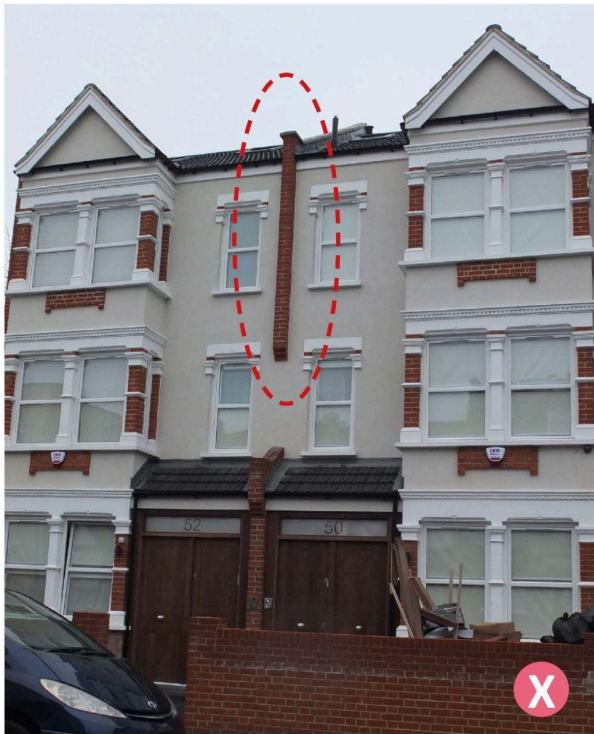
Fig.27: An unacceptable example of a party wall has been corbelled out, not in keeping with the original architectural detailing
